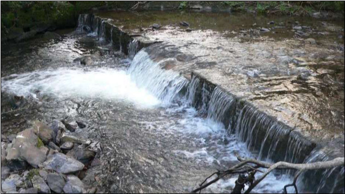
Figure 12: The weir on the River Pulham is a significant barrier to fish passage
