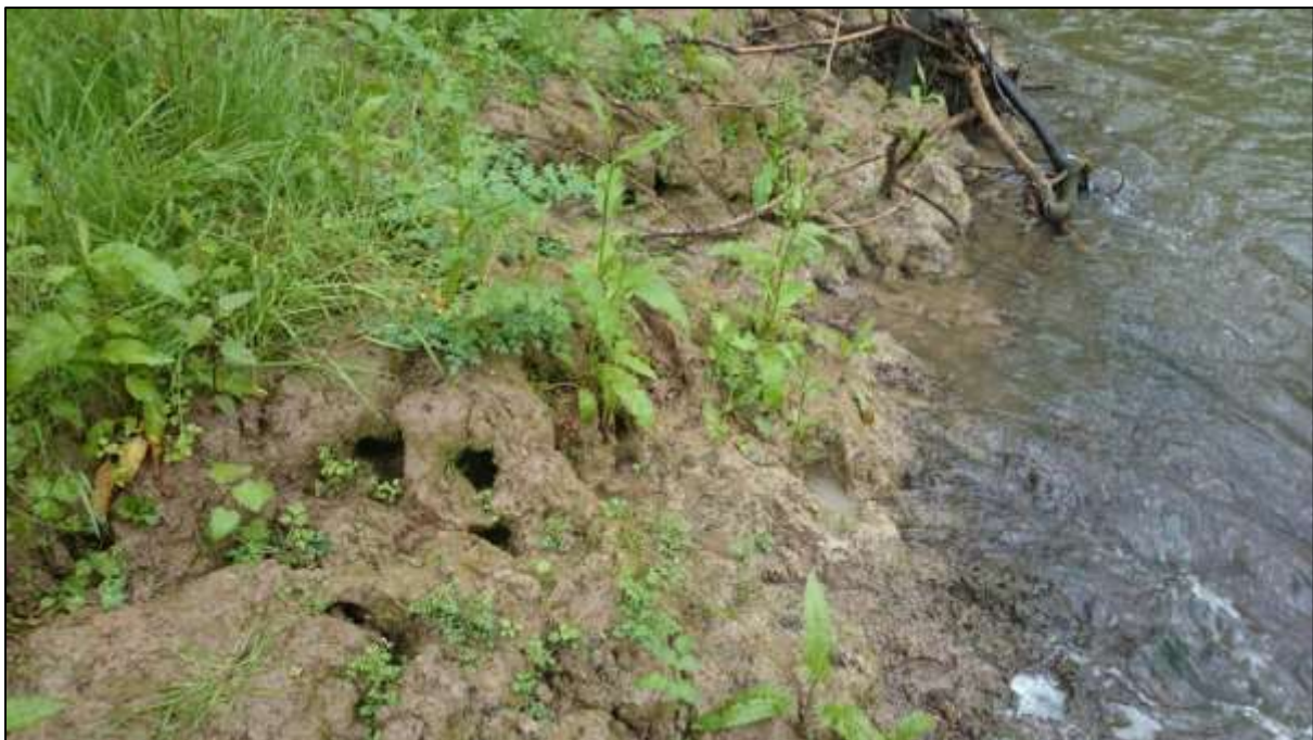
Figure 18: Burrows in the berm at SS 94092 26968 could indicate a signal crayfish infestation
