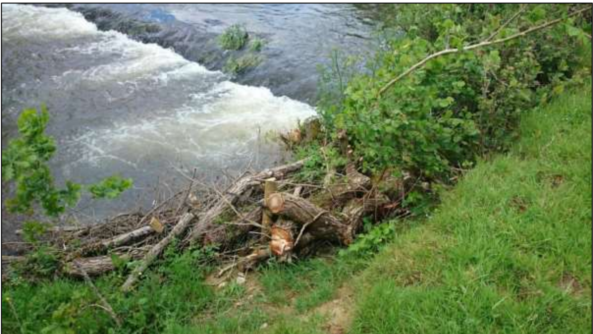
Figure 10: Saplings growing through the bundles will strengthen the bank over time.
