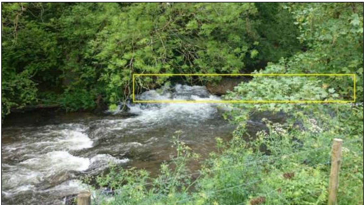
Figure 2: Helebridge Weir (highlighted by yellow box)
